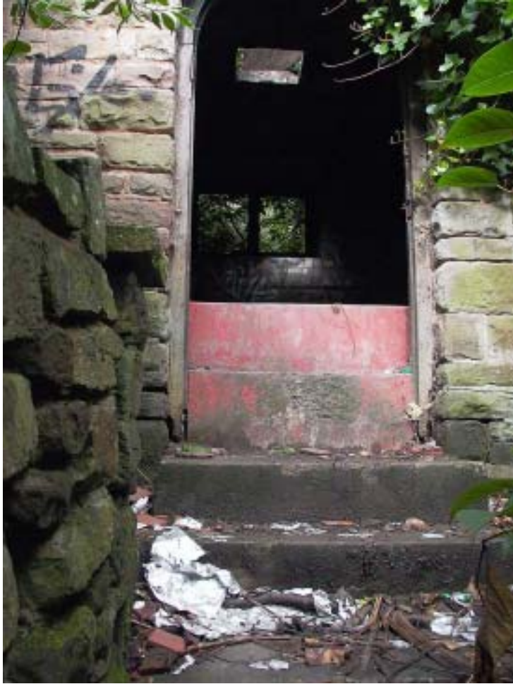
Above: Before - the derelict gas sub-station
